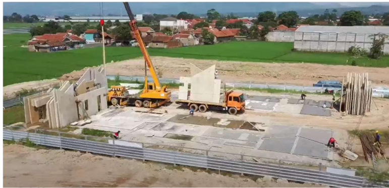
Figure 2. Precast House Panel Production
